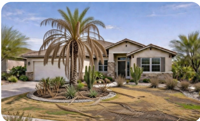
Failure to irrigate with dead plants and debris in the yard.
